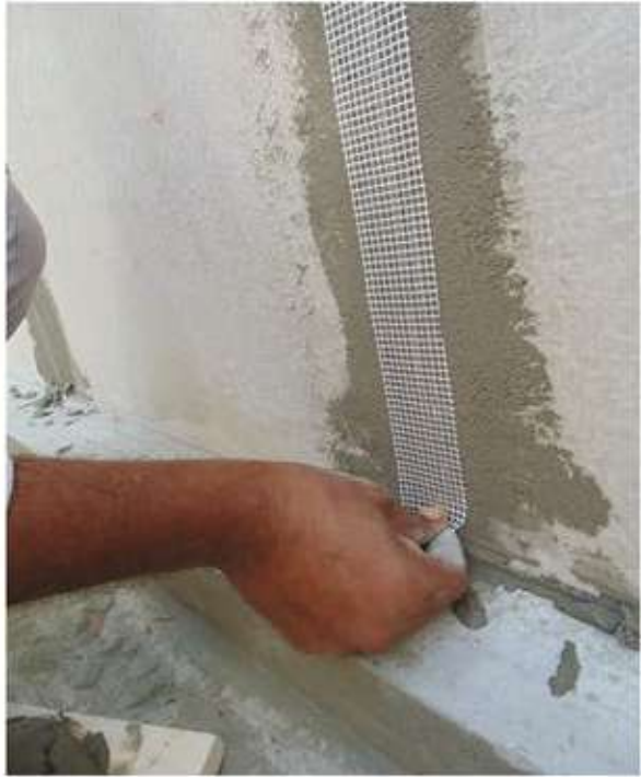
Application of mesh
