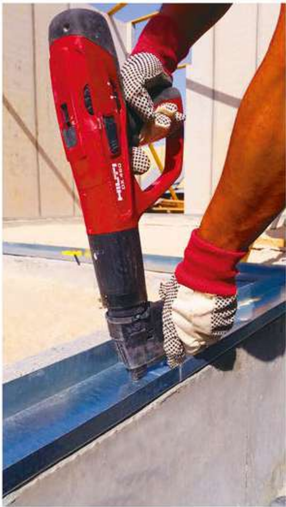
Installation of the base “U” channel
