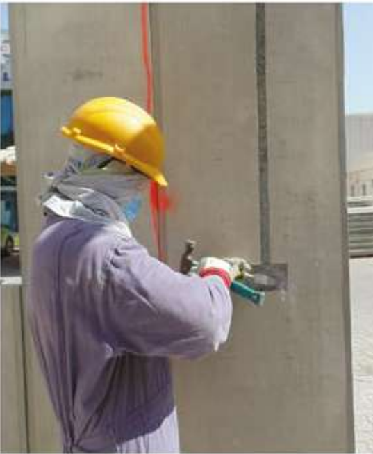
Simple and quick cutouts for electrical conduits
