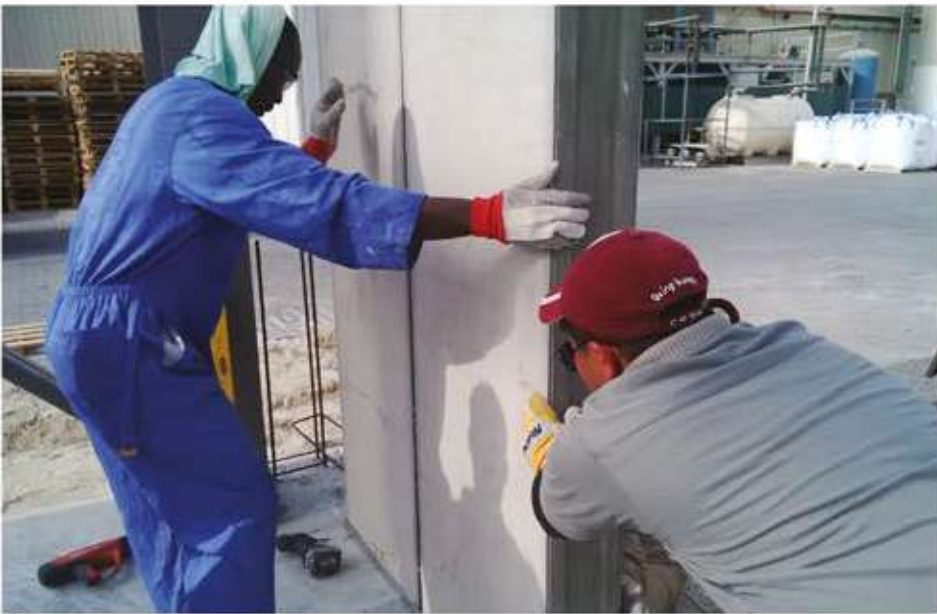
Simple installation of the panels
