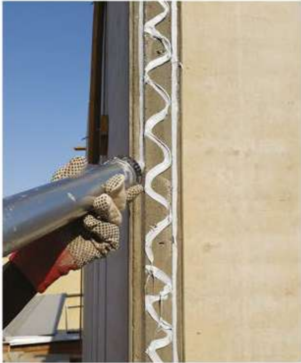
Application of adhesive prior to fixing of panels on-site
